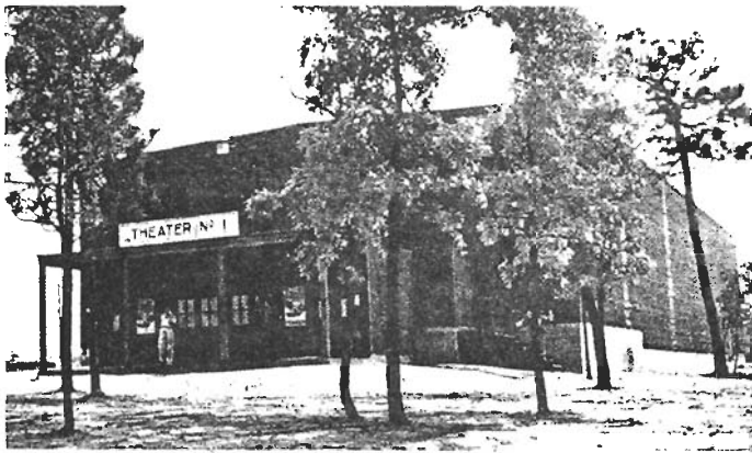
Typical theater, Camp Mackall, North Carolina
