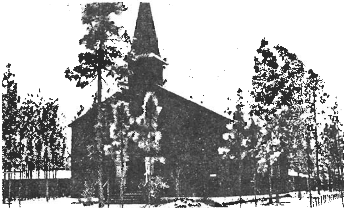
Typical chapel, Camp Mackall, North Carolina
