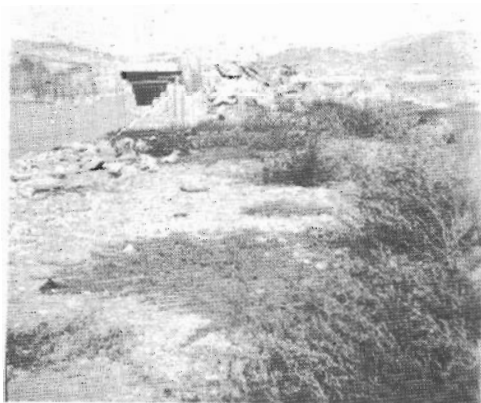
Beach fortification at Nice A demolition job for the 596
