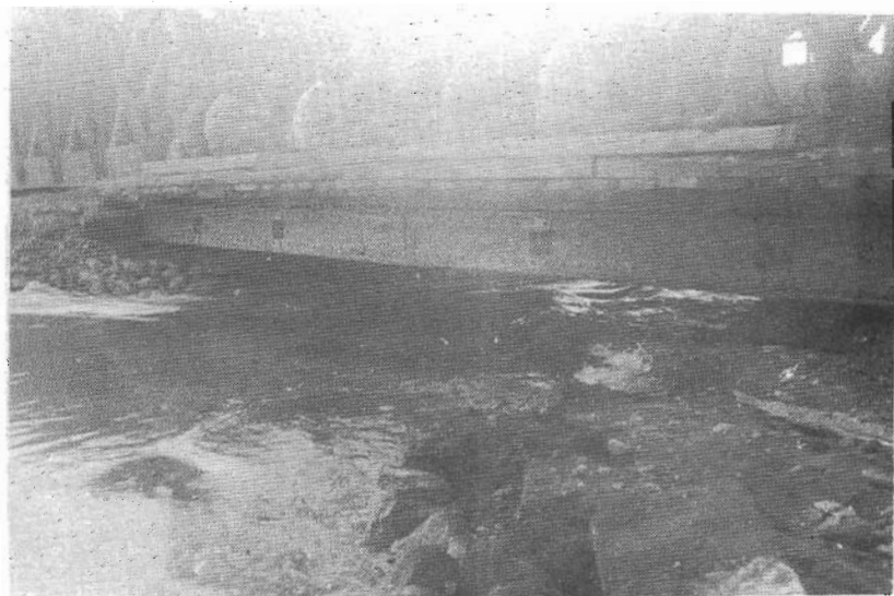
A 596 masterpiece bridge at St. Martin du Var, France
