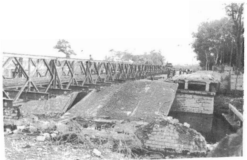
Steel bridge in South of France Did 596 build this?
