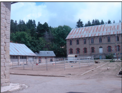
Figure 9. Present day view of a former French Army garrison at Peira Cava.
