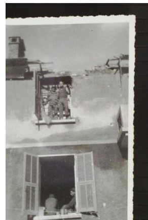
damaged Golf Hotel
