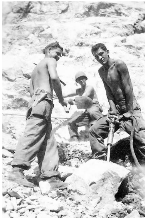
Men of the 1/596 Airborne Engineer repair the Col de Braus road.
